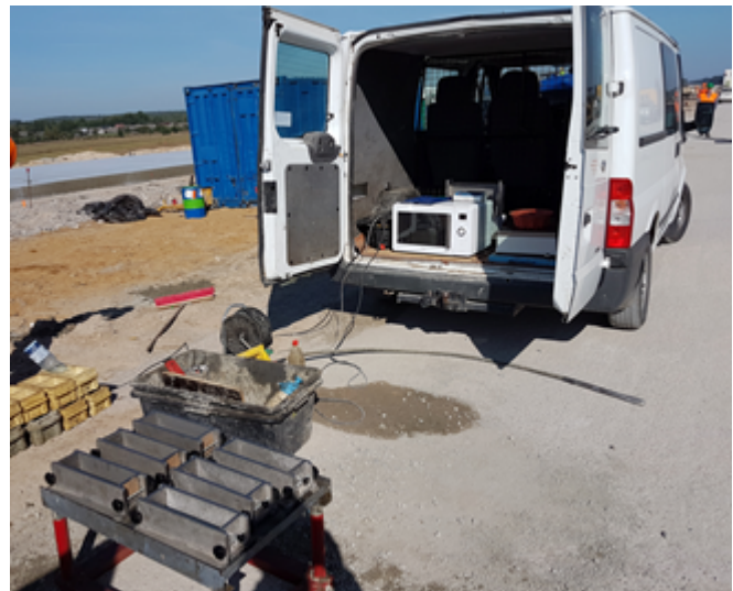
Fig. 1. Field test stand for measuring the water content of the concrete mix by the microwave oven
