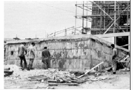
Damage due to liquefaction during the earthquake in Niigata, Japan 1964: Sunk truck (left) and floated up sewage tank (right).
