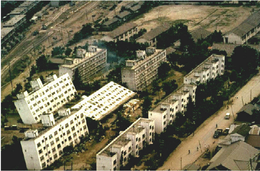
Catastrophic consequences of liquefaction – toppled houses due to liquefaction after the Niigata earthquake, Japan 1964
