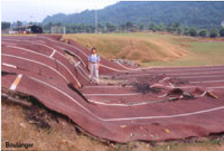
Ground rupture (Taiwan)
