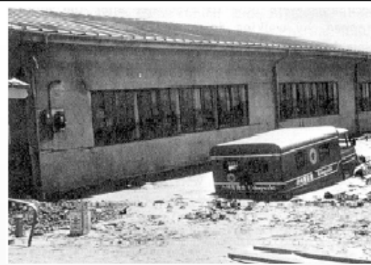
Damage due to liquefaction during the earthquake in Niigata, Japan 1964: Sunk truck (left) and floated up sewage tank (right).
