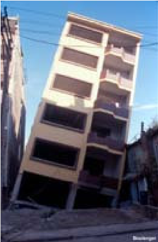
Tilt due to liquefaction (Adapazari)
