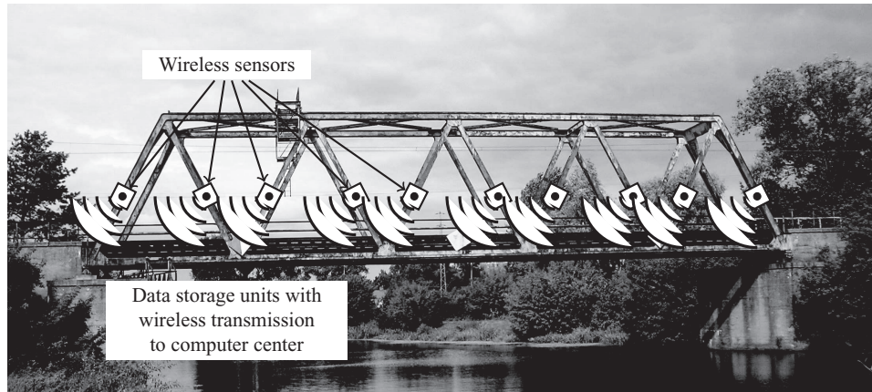
Figure 1.2 A bridge with a wireless SHM system
